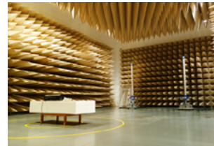
Anechoic chamber used for electromagnetic wave measurement
