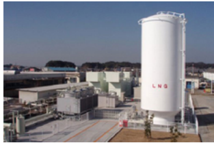
Cogeneration system at Kakegawa Factory
