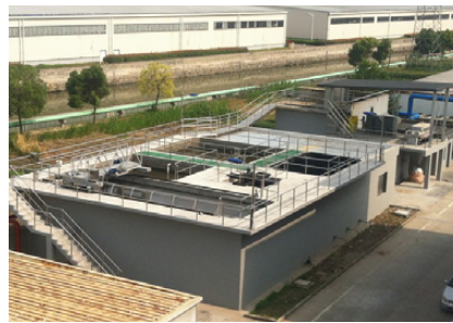
Wastewater treatment facility
