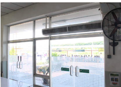
Air curtains for preventing entry by insects
