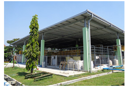
Wastewater treatment facility
