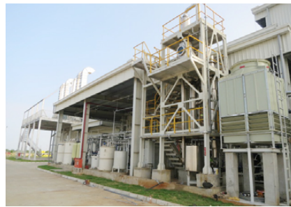
Wastewater treatment facility
