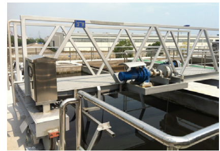
Reuse of wastewater for cooling water
