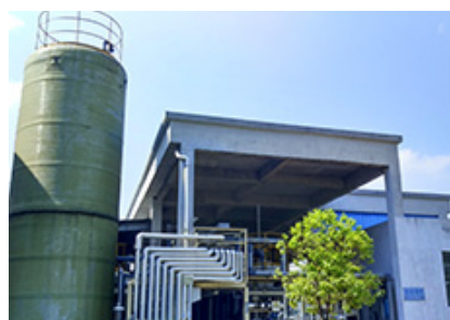
Wastewater treatment facility
