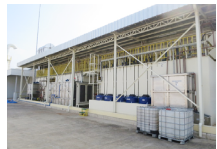
Wastewater treatment facility
