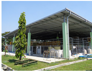
Wastewater treatment facility
