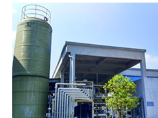
Wastewater treatment facility
