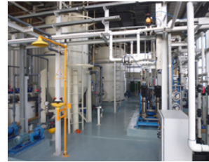
Reuse of 100% of manufacturing process wastewater
