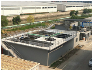
Wastewater treatment facility
