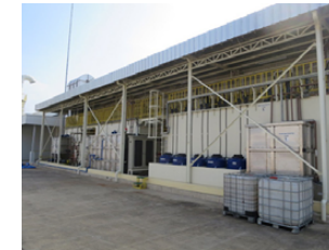
Wastewater treatment facility
