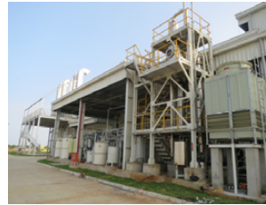
Wastewater treatment facility
