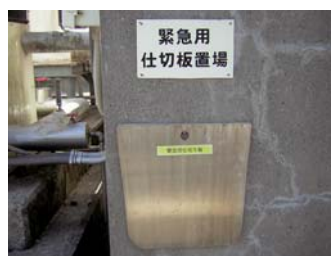
Stopper in case of emergency (Yamaha Kagoshima Semiconductor Inc.)
