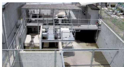
New centralized drain outlet
